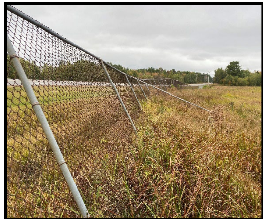
Figure 12. A section of fence at LEW
