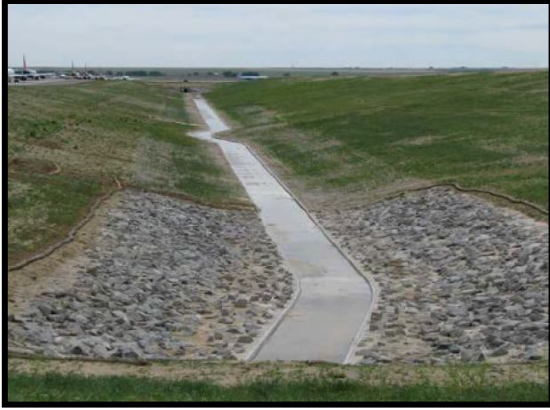
Figure 4. An example of a stream/ditch improvement.
